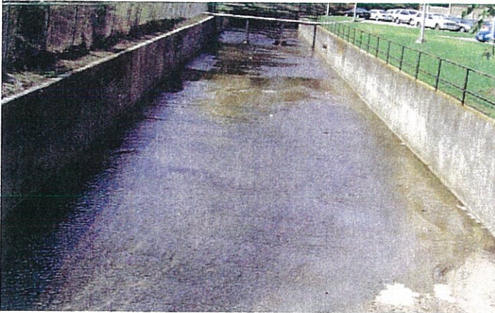
Concrete Flume – Rocky Branch Creek
