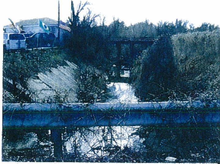
Looking downstream towards Railroad Bridge
