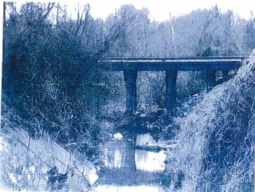
Downstream Railroad Bridge
