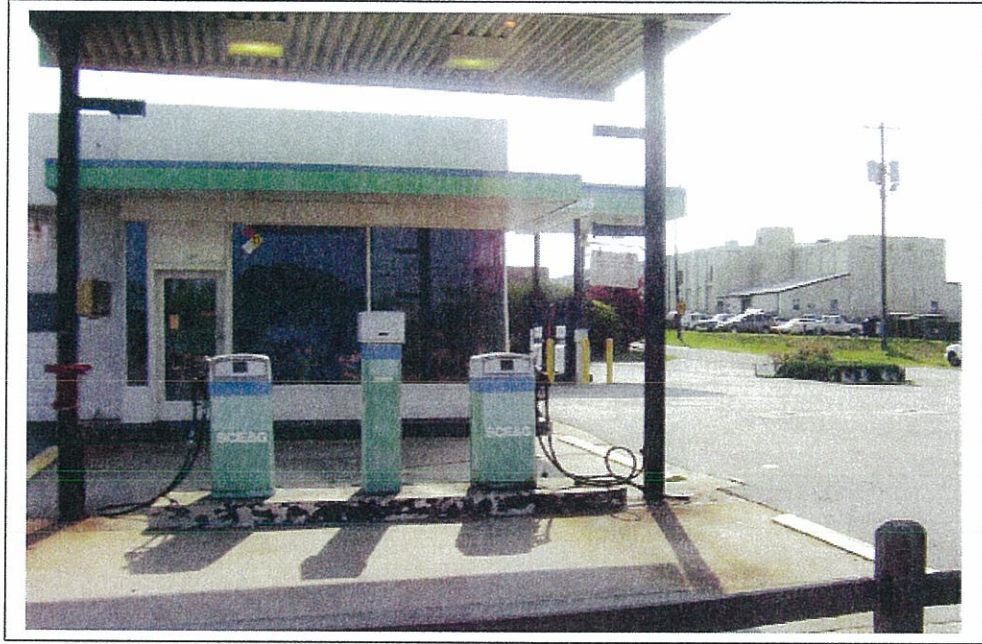
Photograph 3: View of SCE&G Fleet Maintenance at 130 Assembly Street. This facility had a reported LUST and has a no further action date of November 10, 1992. These pumps shown are listed as currently inactive
