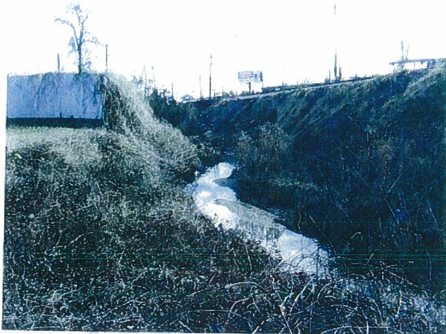
Upstream looking Downstream toward Rocky Branch
