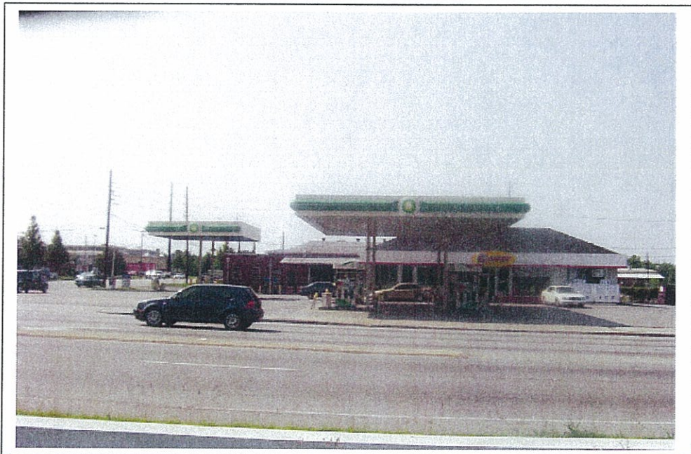
Photograph 8: View facing south of BP Gas Station in southwest corner of Blossom Street and Huger Street intersection near the project area boundary. This facility is currently in operation.
