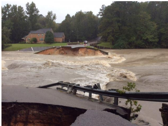
Carys Lake Dam failure
