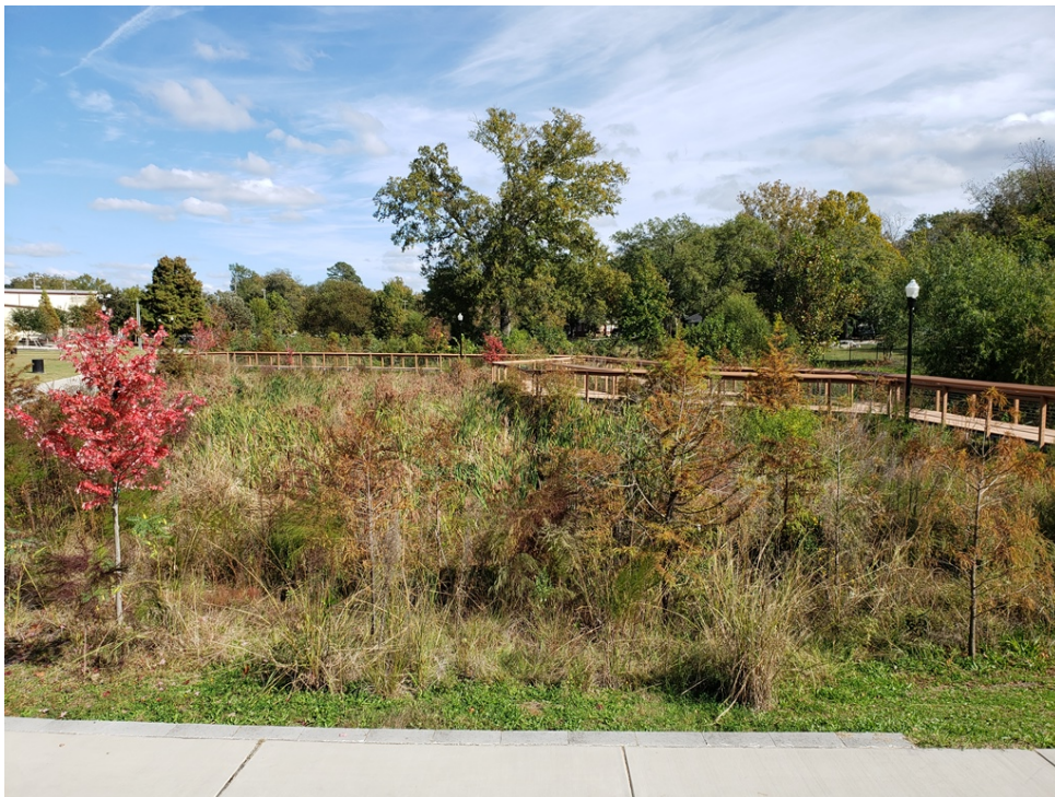
Figure 6. Detention basin adjacent Rocky Branch in Martin Luther King Junior Park in November 2020.
